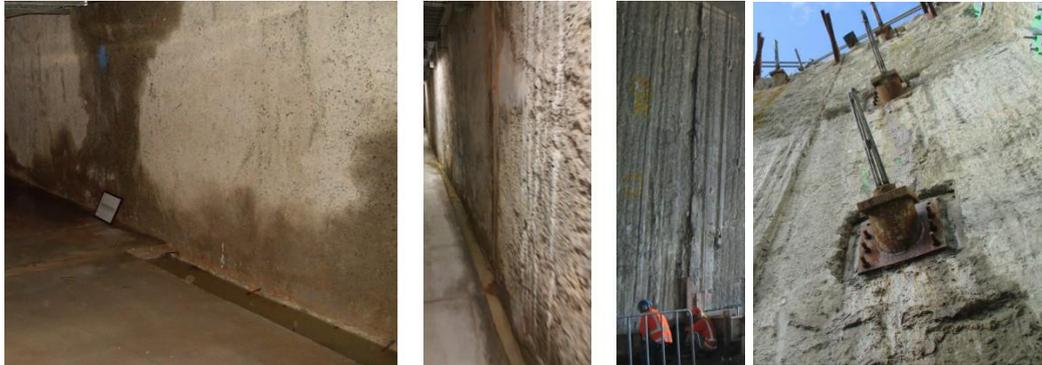
Figure 4. Selected narrow diaphragm walls constructed in soil conditions with high ground water tables showing minor damp patches, thus providing adequate 'water tightness'
