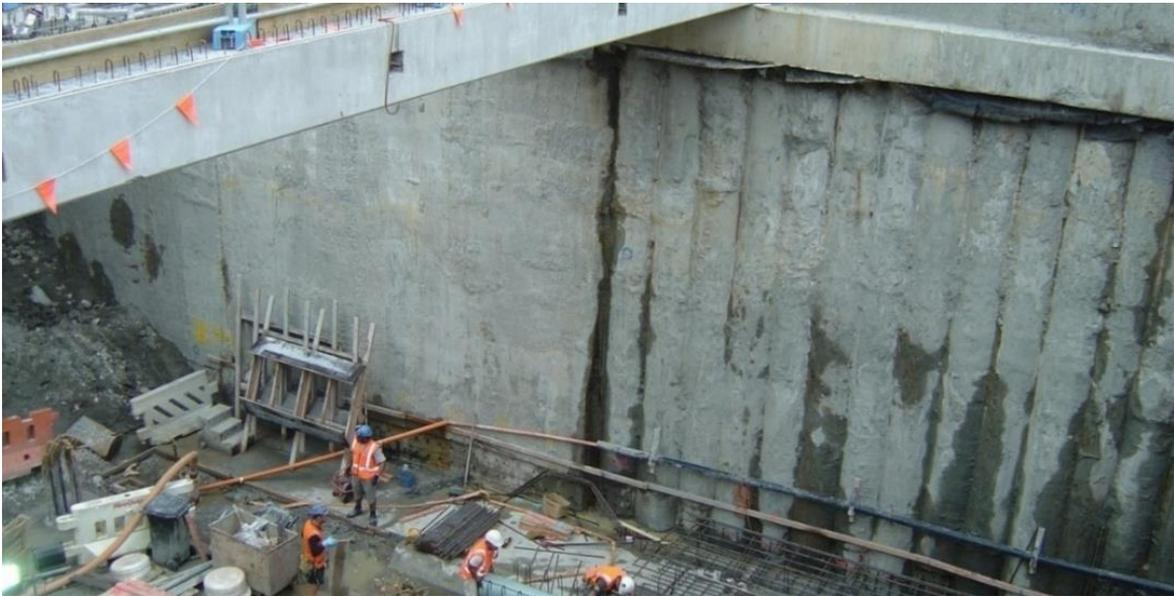
Figure 1. The diaphragm wall section (left) has fewer vertical joints per m<sup>2</sup> of wall surface, which provides superior water proofing performance than the secant pile wall section (right)
