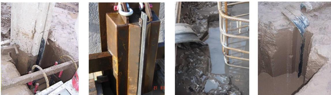
Figure 3. Different ‘stop-end’ profiles showing varying profiles with the purpose to extend the potential flow path of water along the joint (left). Water-‘stops’ are installed inside the joints.
