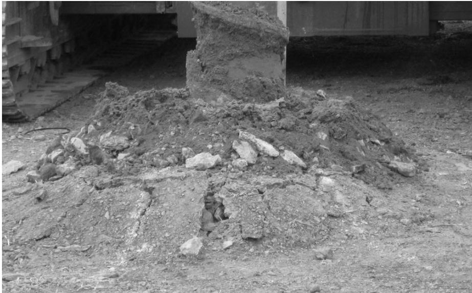
*Figure 5. Ground heave occurring during the installation of test pile E (axis B-B)*
